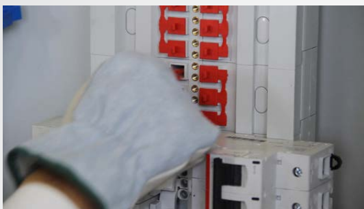
The Protective Cover Is Removed
