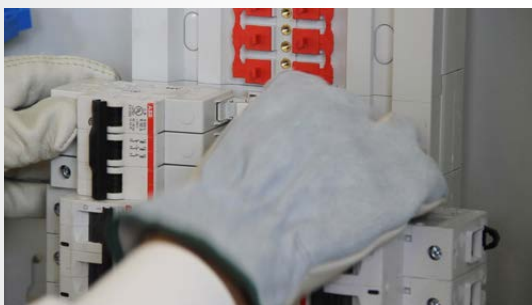
The Breaker Snaps Into The DIN Rail
