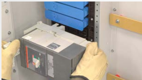
The Breaker Is Inserted Into The SafePanel
