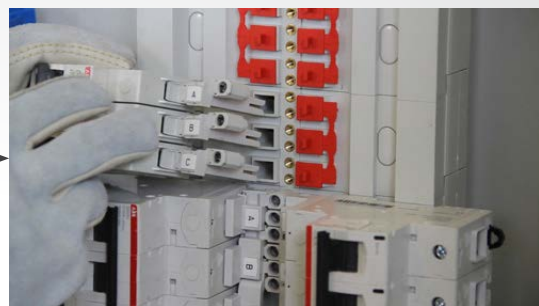
The Breaker Is Inserted Into The Opening
